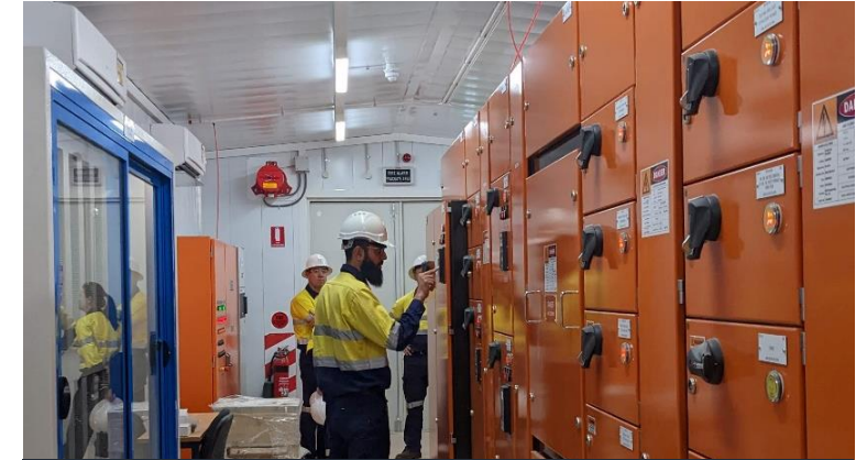
HV Infrastructure Upgrade (2023)
